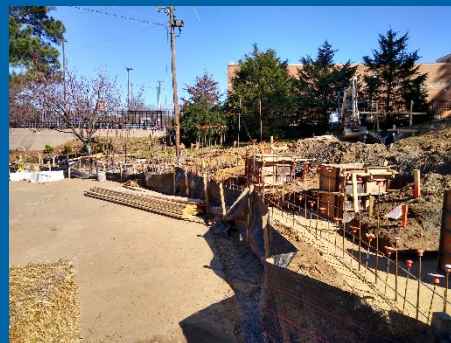
Continue excavation of canopy footings and retaining wall and pouring concrete
