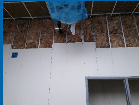
Insulate metal studwalls and hang 2 nd side of drywall
