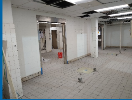
Prepare Kitchen Floor for Epoxy Floor Application
